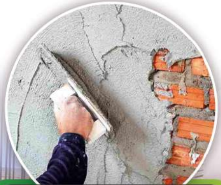
Plastering Works
